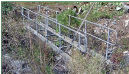
Sewage works infrastructure before remediation
